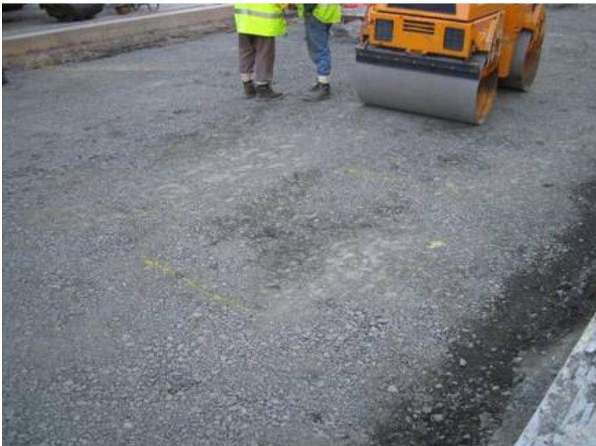
Figure 11 Soft Spots Identified from LWD Testing, Marked Up On Site and Undergoing Proof Rolling
